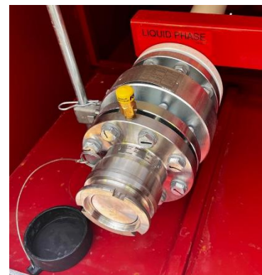
Figure 9 - Example of MannTek male adapter Dry Disconnect Coupling with Rego safety valve (courtesy of MannTek and Rego)
