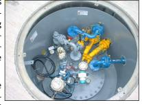
LPG. Wherever possible, only one connection, excluding the drain line, should be provided and all the rest should terminate in the vapour space.
