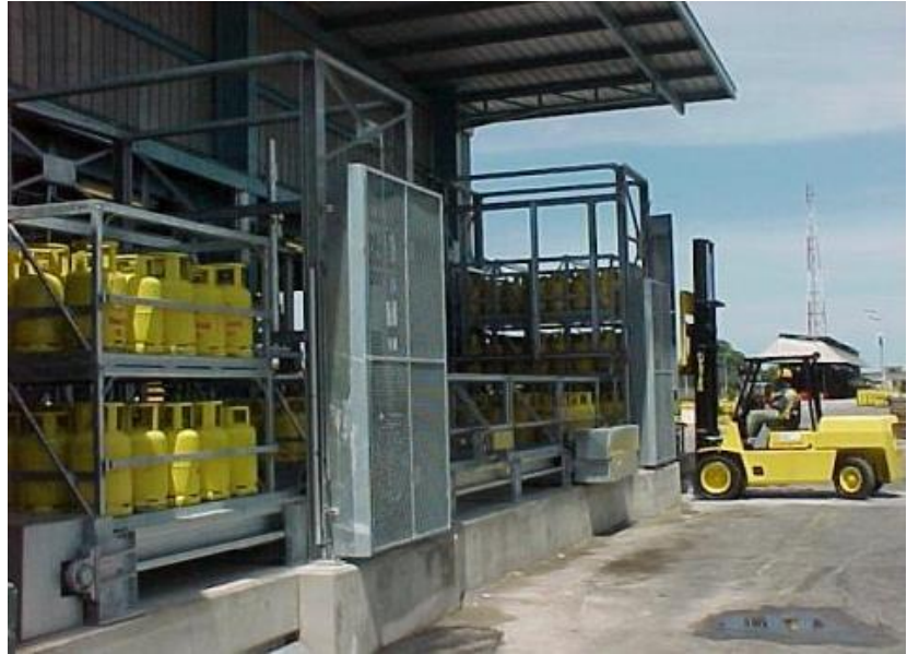
Example of a palletising system
