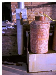
These cylinders have been placed in a hot water bath to assist vapourisation but this will accelerate corrosion
